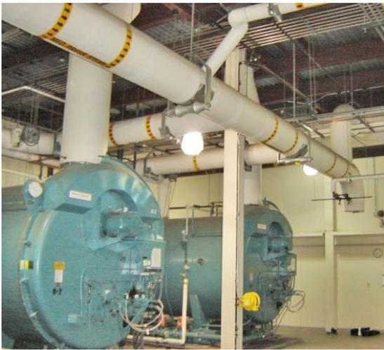
**Figure 2 – Boiler header in a healthcare facility**
