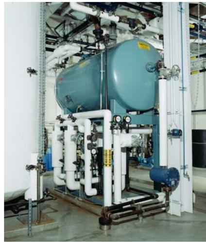
**Figure 4 Deaerator (DA) tank in boiler room**
