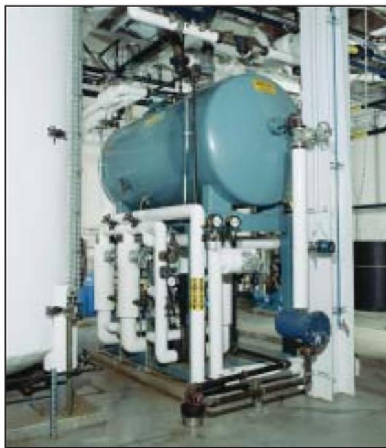
**Figure 3:** Deaerator (DA) tank in boiler room
